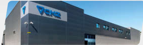
CENTRAL SERVICES | TECHNICAL ASSISTANCE SERVICE Zaldibar – Spain
