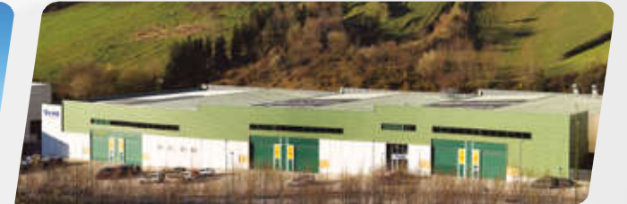
CNC lathes Assembly plant 10,000 m2 | Mallabia – Spain
