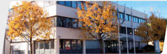
COMMERCIAL OFFICE | TECHNICAL ASSISTANCE SERVICE Stuttgart – Germany
