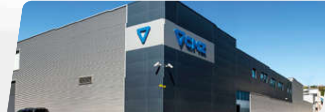
CNC lathes Assembly plant 5,500 m2 | Zaldibar – Spain
