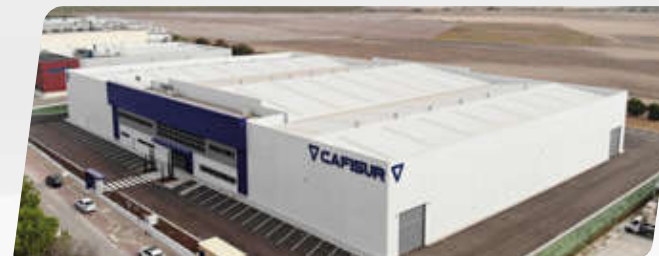
Sheet metal plant 15,000 m2 | Cádiz – Spain
