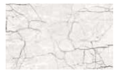
FCS 547 Cracked marble
