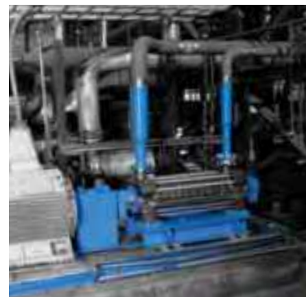
Adjustment reducers & retrofit base frame
