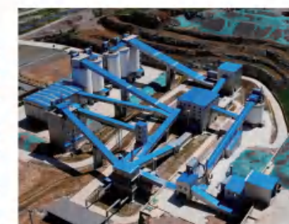
砂石骨料生产线 Sand and gravel aggregate production line
